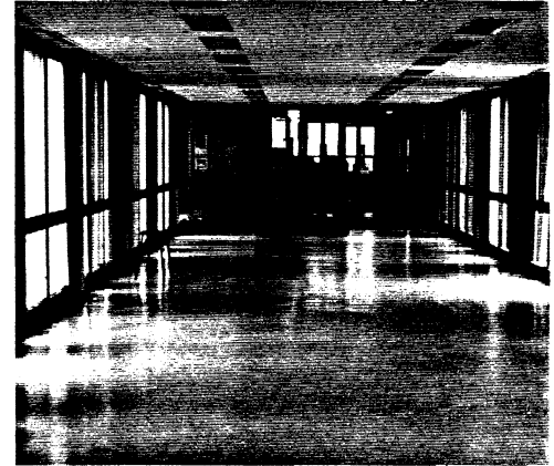
Corridor with parallel glass side walls. Glass is highly reflective in the mid and high frequencies.
